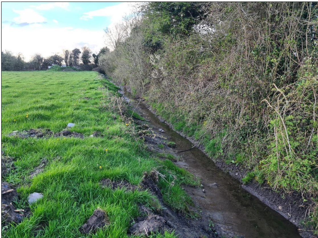
Plate 2-24 Drainage ditch (FW4) and treeline (WL2) located between fields for the proposed end masts.
